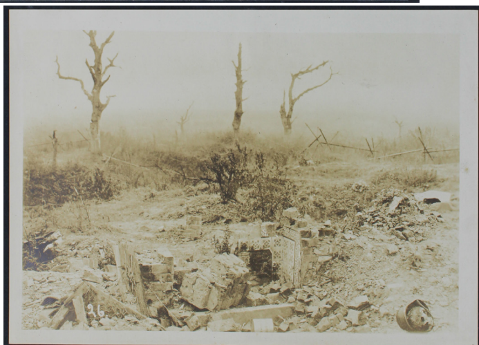
26. NO MAN'S LAND...The only recognizable thing left in the city, the remains of a fire-place. Looking South across the terrain, which until the American Drive had been No Man's Land since 1916. Note the barbed wire and what was left of a "Jerry", Haucourt, near Malancourt, Meuse, France, November 7, 1918.
